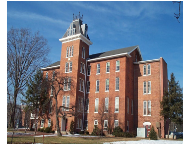
Juniata College Founders Hall Additions & Renovations Huntingdon, PA
