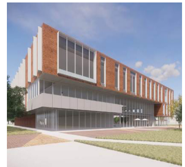
Ohio University (HCOM) Phase I Expansion Athens, OH
